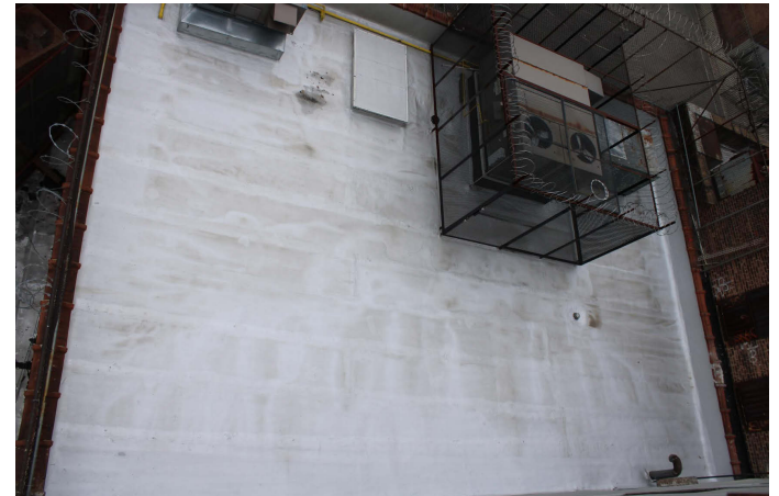
Adjacent Roof Access
