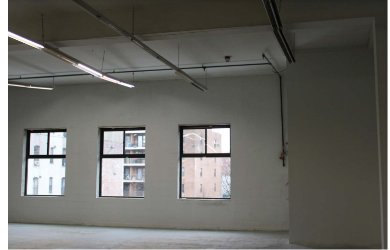
View to Rear of Building
